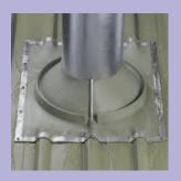
Where damming is a risk and there's difficult access, use a Dektite \*Retrofit \*Soaker \*Just wrap it around the pipe and crimp it.
